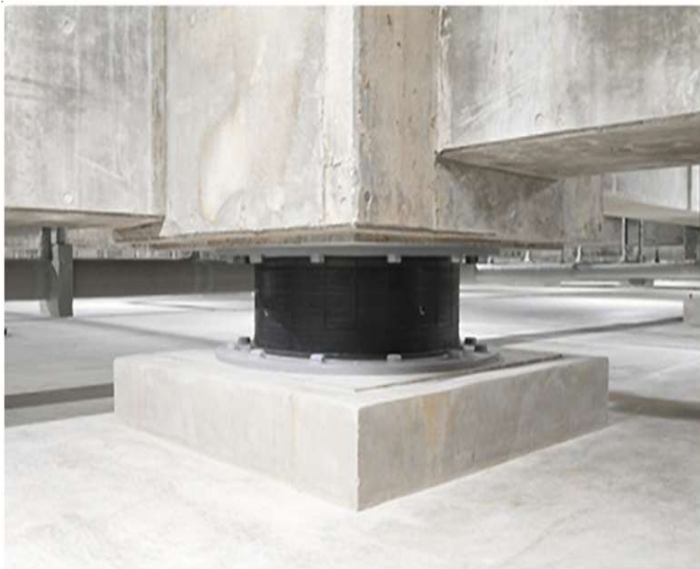
Figure 1 Base Isolated Building
